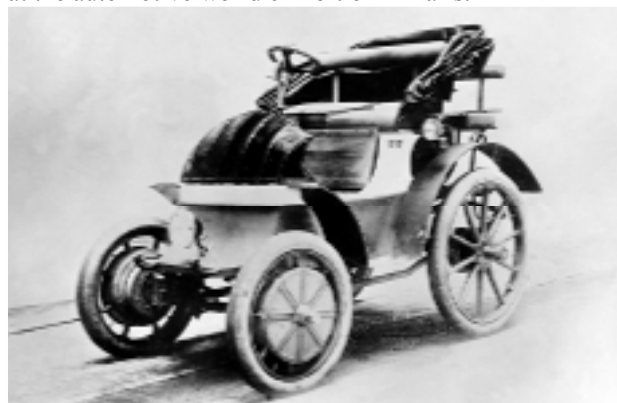
Fig.1. Lohner-Porsche battery driven electrical vehicle [2]
